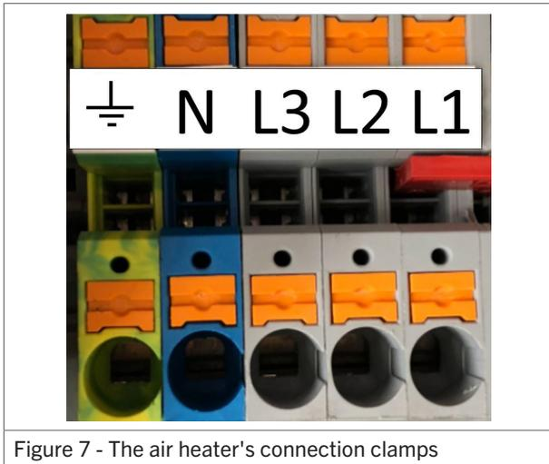
Figure 7 - The air heater's connection clamps
